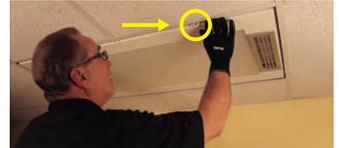
**NOTE:** Use protective eye wear and gloves while you are handling the MERV 6 filter. Use proper disposal instructions for hazardous waste materials.
