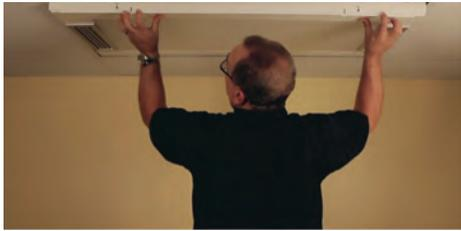
**CAUTION:** It is best to perform maintenance when the power to the VidaShield is completely disconnected. Always wear eye protection and do not look directly at the UV light.
